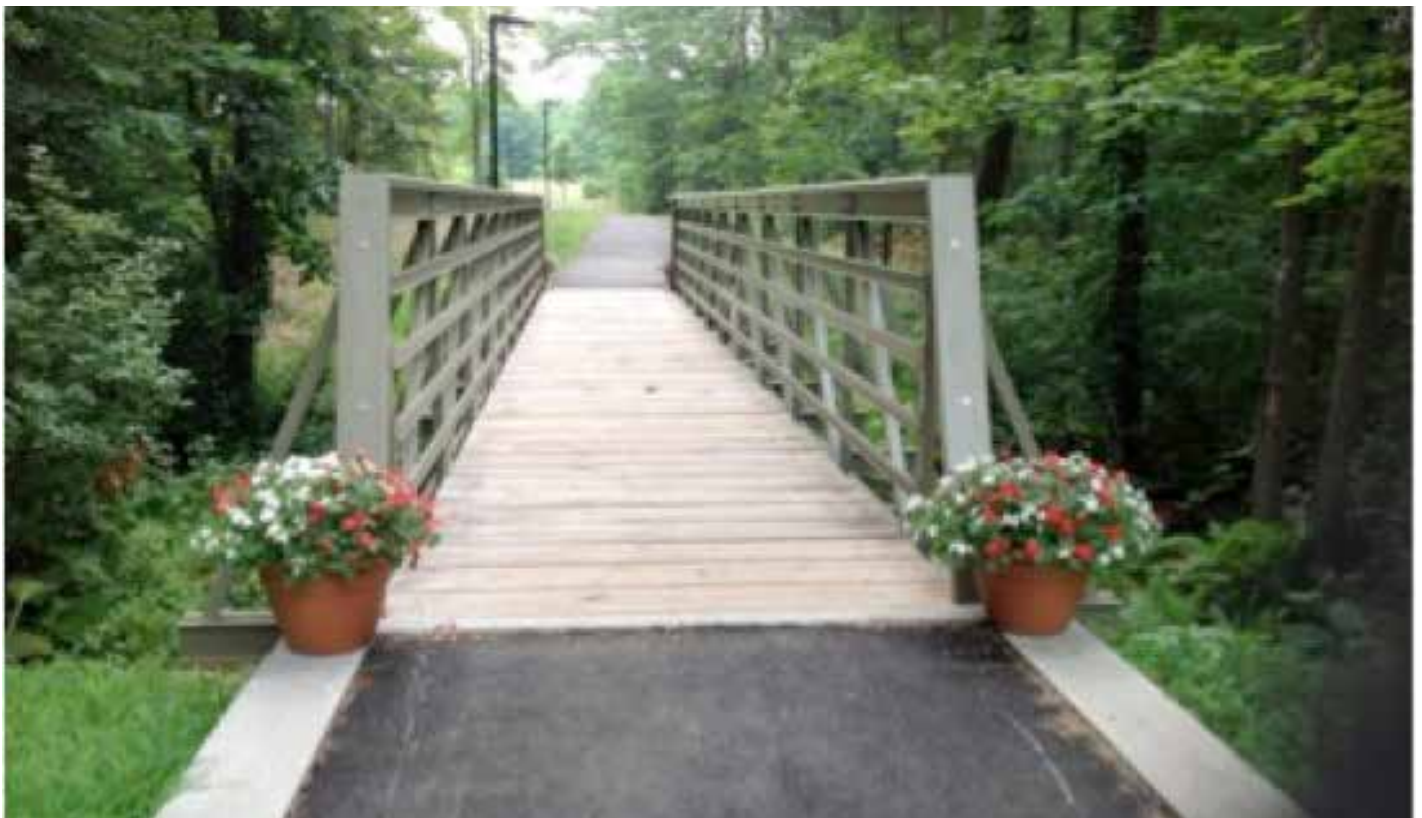
Boxborough's innovative fiberglass pedestrian bridge
