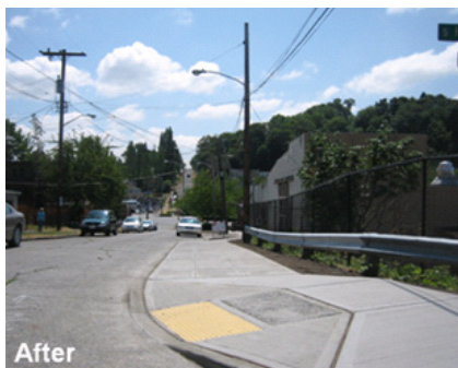
New sidewalk along 39th Avenue South in Southeast Seattle. Source: Seattle DOT
