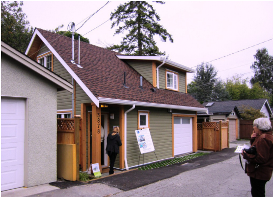
Laneway homes in Vancouver, BC, replace traditional garages and face onto an alleyway. Source: Michael Geller
