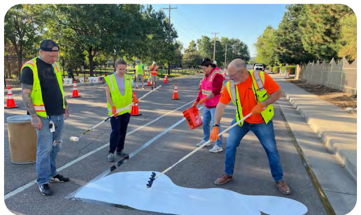
Volunteers prepare the asphalt with primer (Wheat Ridge, CO)
