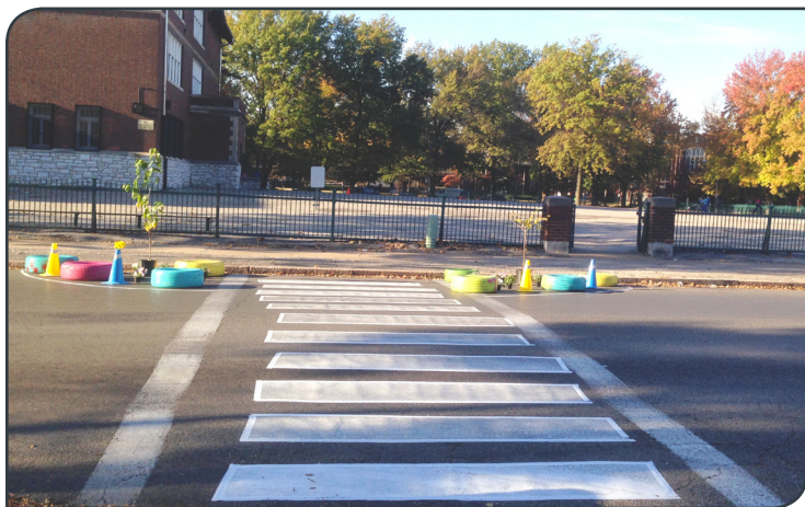
This pop-up crosswalk draws attention to where people will be crossing the street. The traffic cones and colorfully painted tires are arranged as a curb extension, which narrows the road in order to slow traffic and shortens the crossing distance for people walking. Photo: TrailNet
