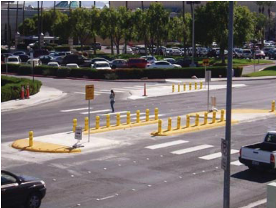
Offset crosswalk with high visibility crosswalk markings in Las Vegas, NV. Source: Federal Highway Administration, United States Department of Transportation
