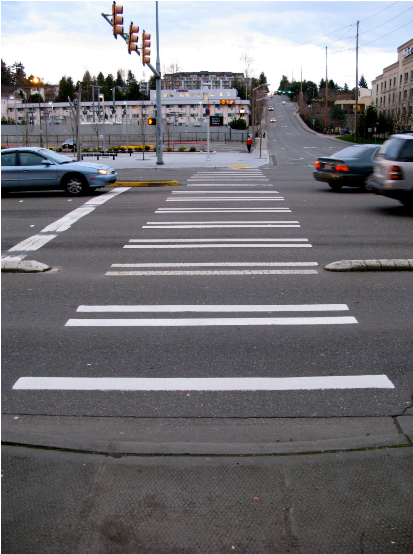
Bar-pair high-visibility crosswalk markings across International Boulevard in SeaTac, WA. Source: Oran Viriyincy, Flickr
